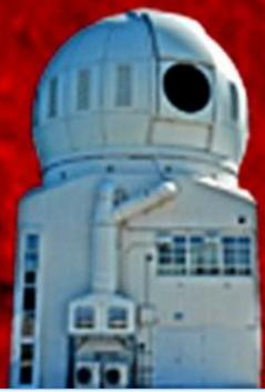
**The NST is an off-axis Gregorian telescope with a 1.6 meter primary. A field stop at prime focus rejects most of the solar light allowing a field of view of 120 arc-seconds.**
